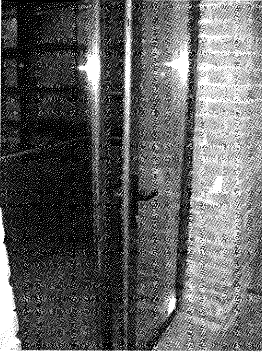
Figure 3: The balcony doors when opened for the ajar measurements to simulate the need for airflow.
